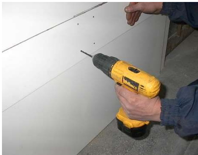
9 – make a small pilot hole at all 12 fastening points. When finished remove template
