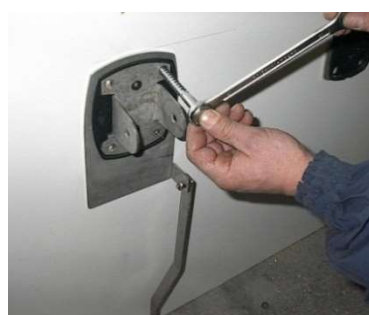
10 – attach flange securely to the wall use photo 12 as a guide
