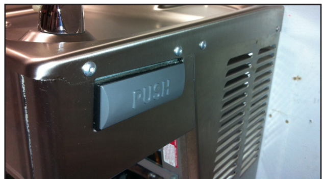
Fasten Basin Assembly in place.
